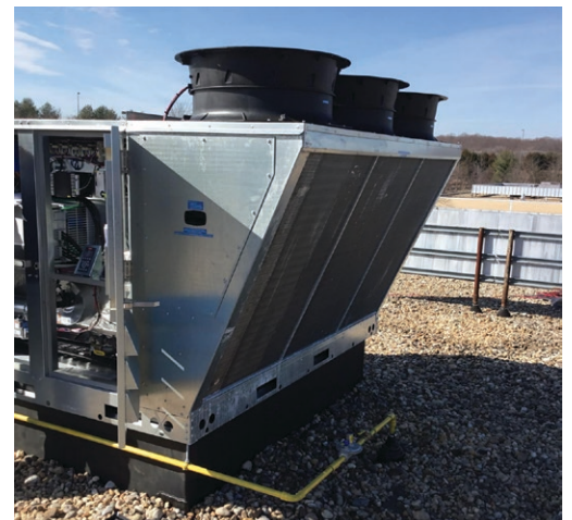
RuppAir's HVAC Unit Installed at the Laboratory
