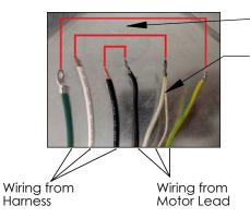
SO/SJ Cord from disconnect is wired to the ECM wire harness and motor wiring in speed control handy box.
