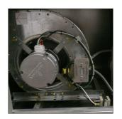
4 Pin communication connector from the EVO/ECM is connected to the ECM motor.
