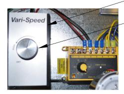
Handy box part number 58371-1/2 is installed on the electric board. The handy box is installed on the lower left corner when possible.
